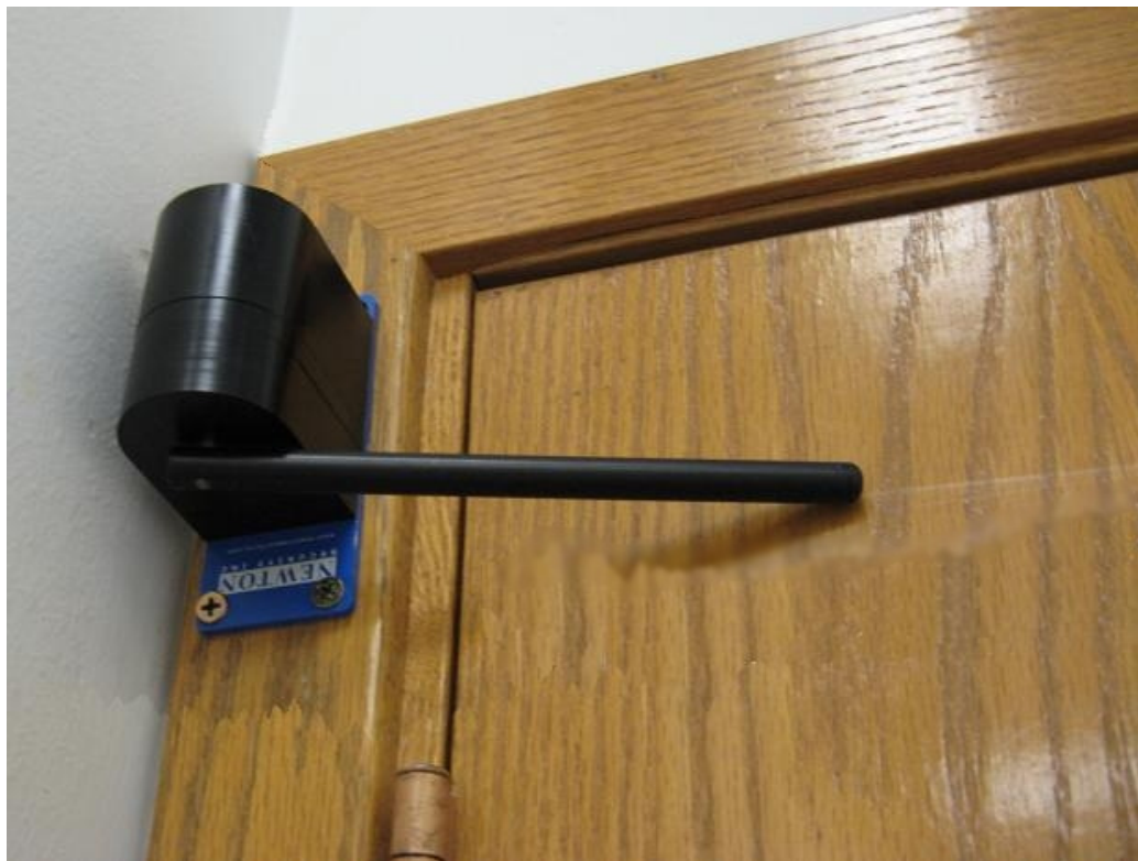
Figure 39 –Position of Encoder (Public door only)
